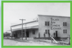
SASCU Opens. Works outside of Farmer's Exchange
